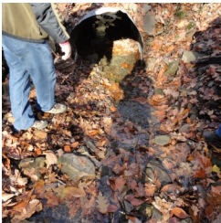
Undersized pipe on Dark Hollow, Gibson Township
