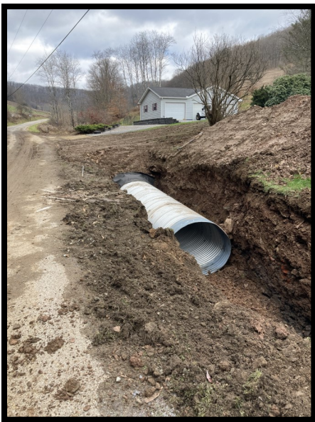
Plank Road Hollow Pipe Replacement
