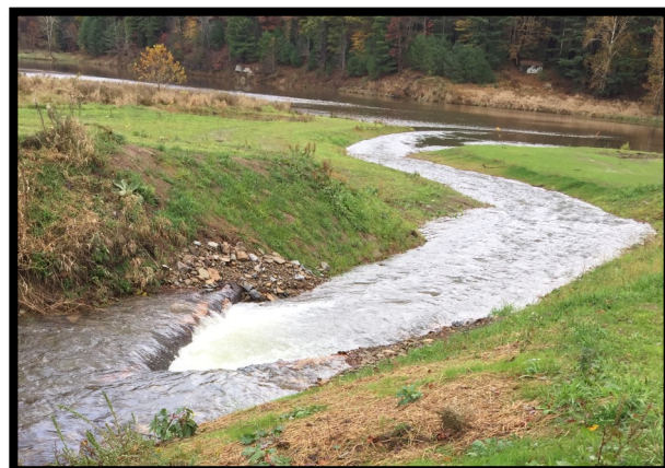
Crossvane installed in Brooks Run, that leads into George B. Stevenson Dam.
