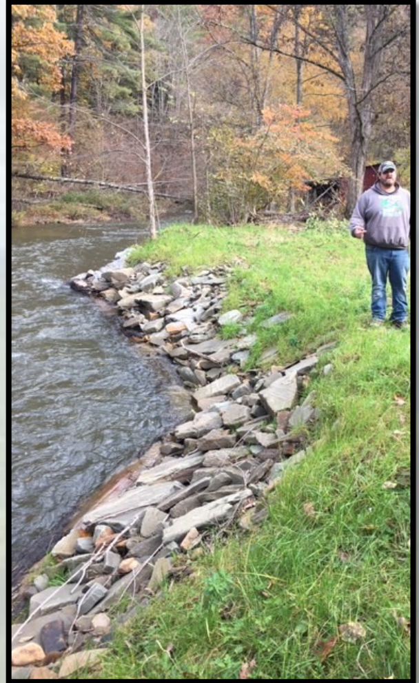
The Grovanz Stabilization Project that was completed in 2018.
