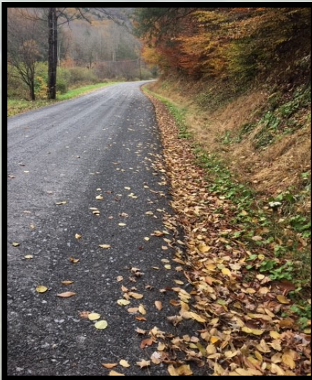
Shippen Township, Sizer Run project 3,400' of DSA installed.
